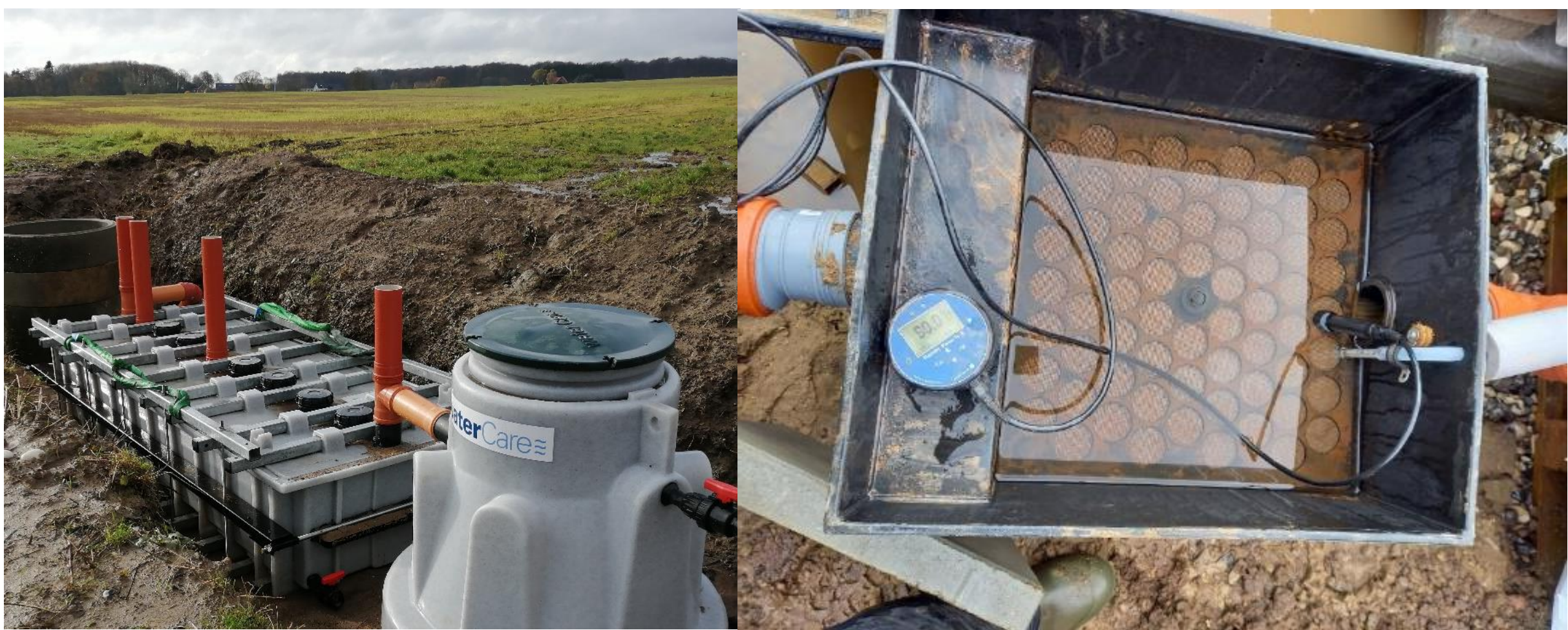
Figure 2: Sediment filter (left) and reactive filter (right)
