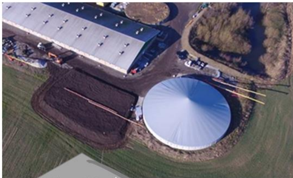
Gylletank tank 4400 m 3
